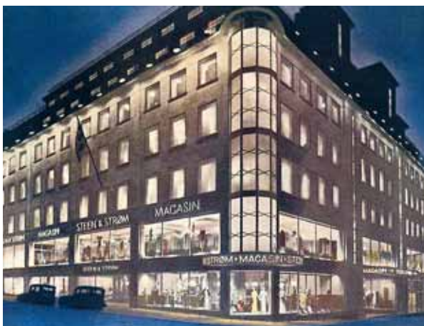
Steen & Strøm Magasin in 1930, rebuilt after the fire.
